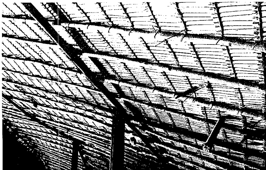
FIGURE 6.—Detail of the thatch at Watoriki . Note the slender Socratea wood slats around which the individual leaves are folded, visible at the top right of the picture. Each leaf is folded double at the midrib (at the edge furthest from the camera).
