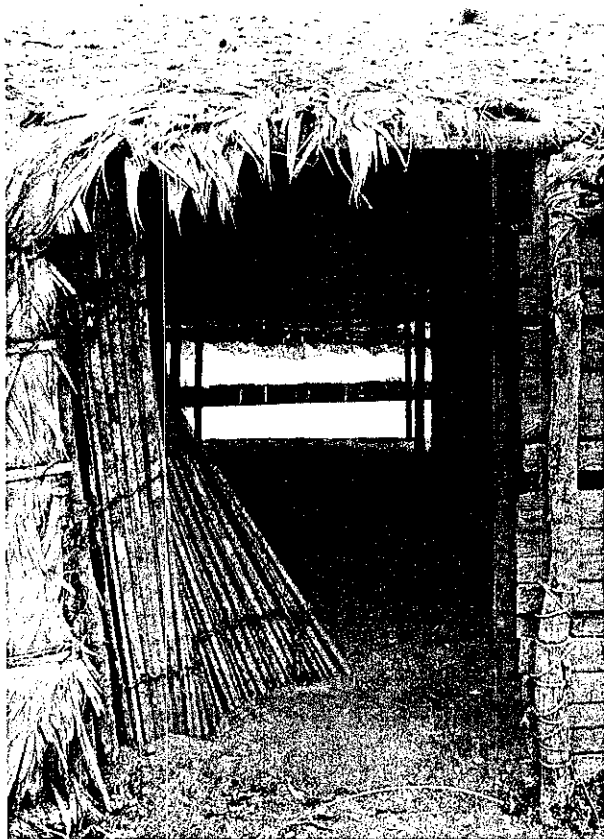
FIGURE 3.—Detail of one of the main doors ( pata yoka ) at Watoriki , looking inwards. Note the thatched wall on the left, the Socratea -wood wall on the right, and the folding door (also made from Socratea wood).
