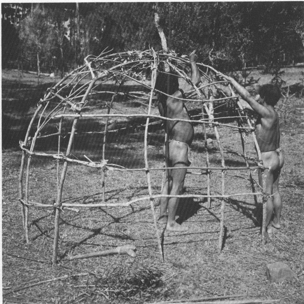
FIG. 12. Building a tapuy framework; tying the horizontal sticks on the vertical poles.
